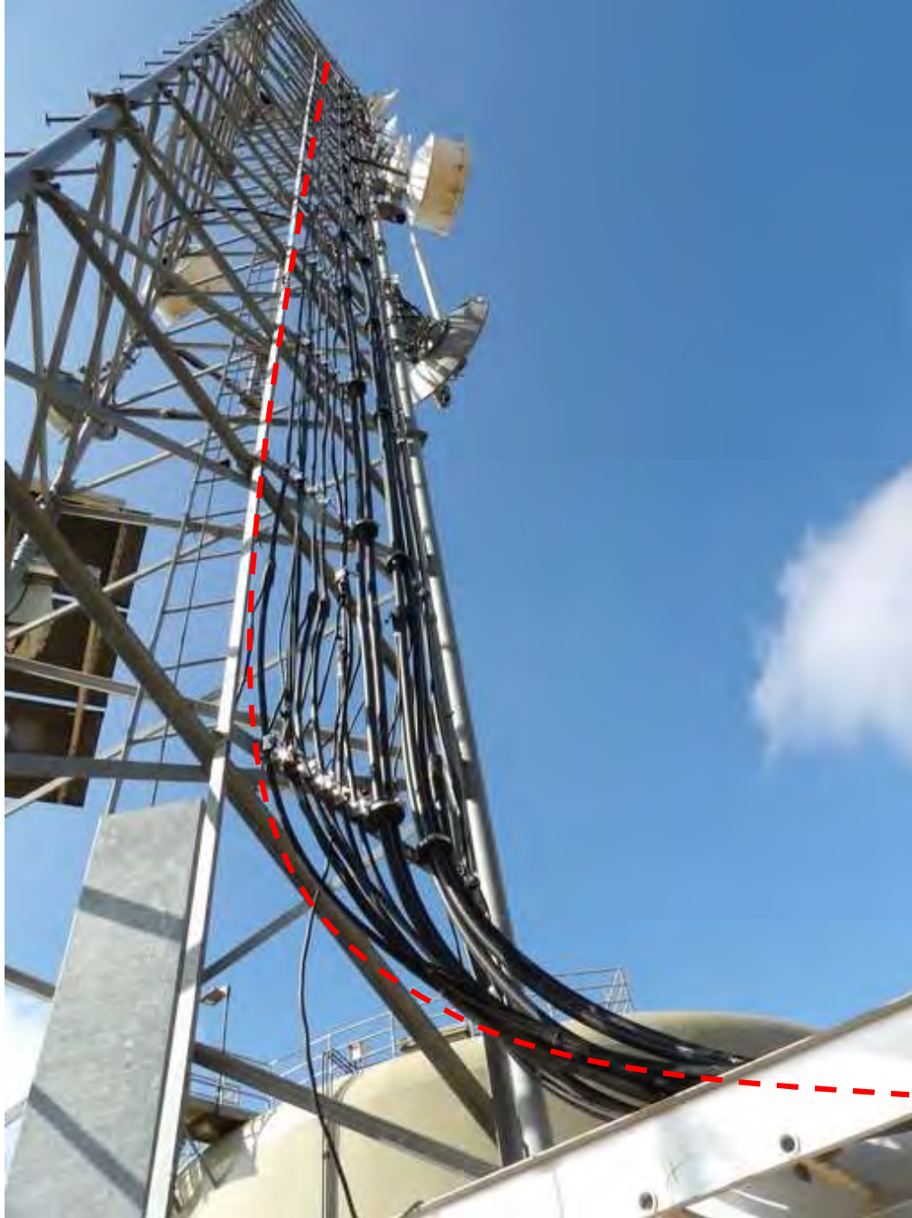
Antenna Waveguide Photo
