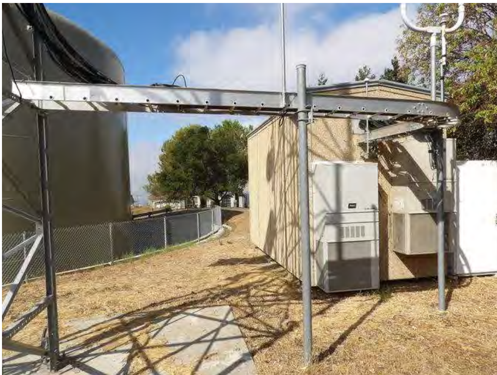
Antenna Cable Ice Bridge
