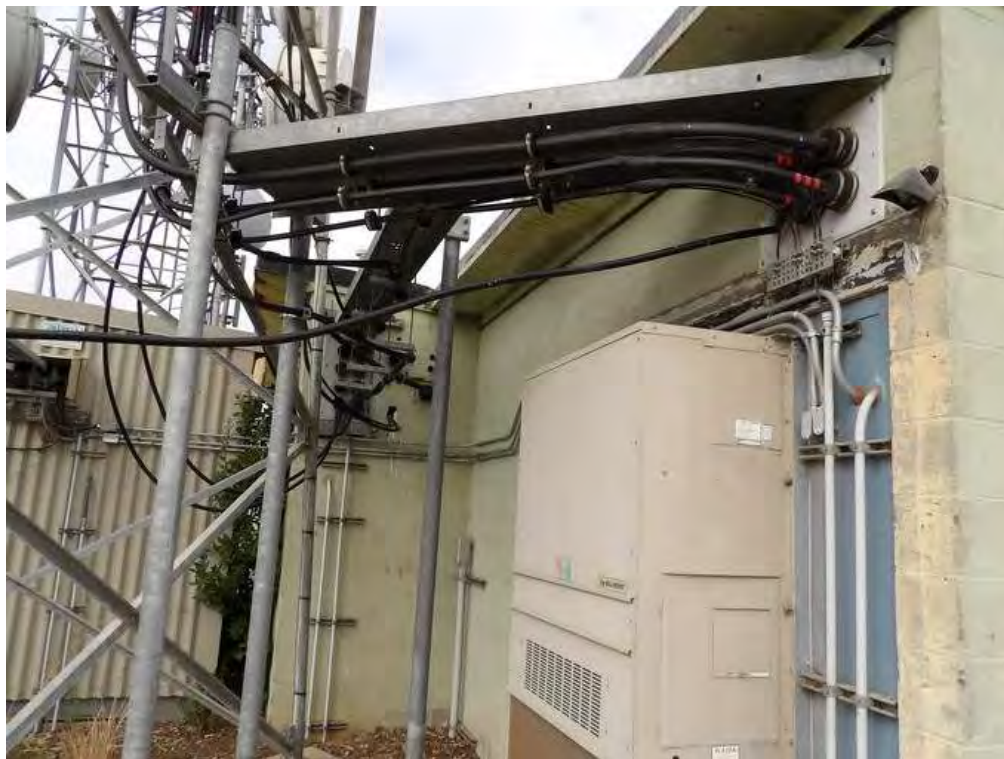
Antenna Cable Ice Bridge
