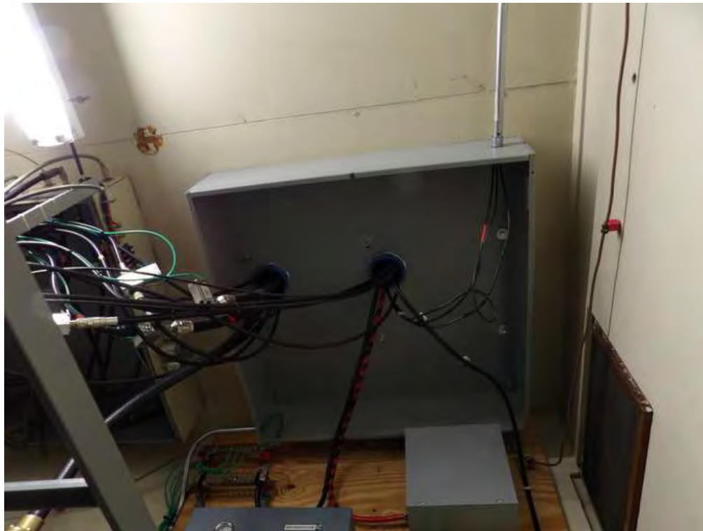
Antenna Interior Entry Port
