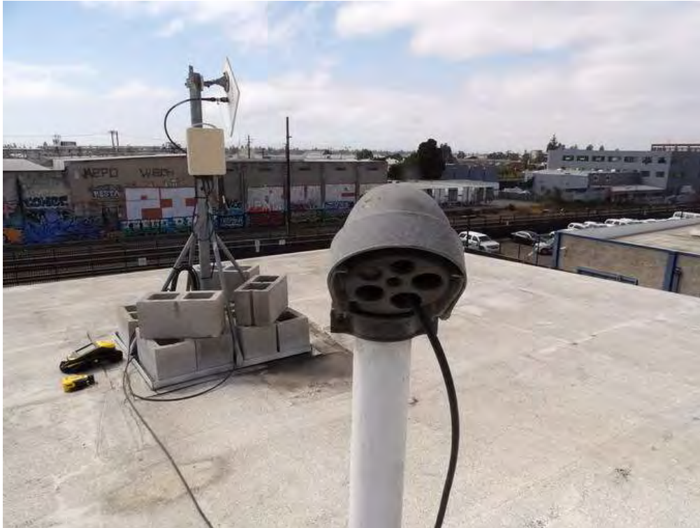
Antenna Cable Exterior Entry Port
