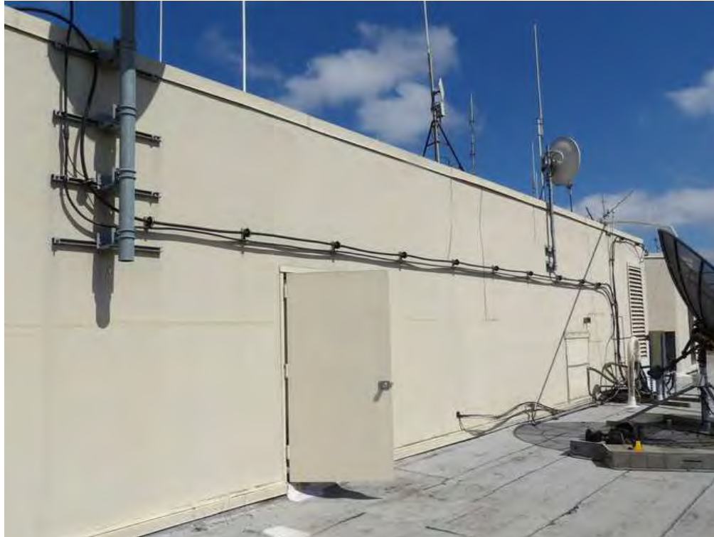
Antenna Cable Ice Bridge
