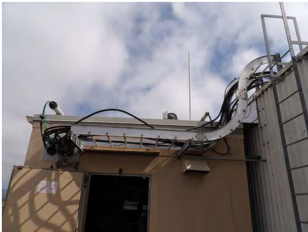
Antenna Cable Ice Bridge
