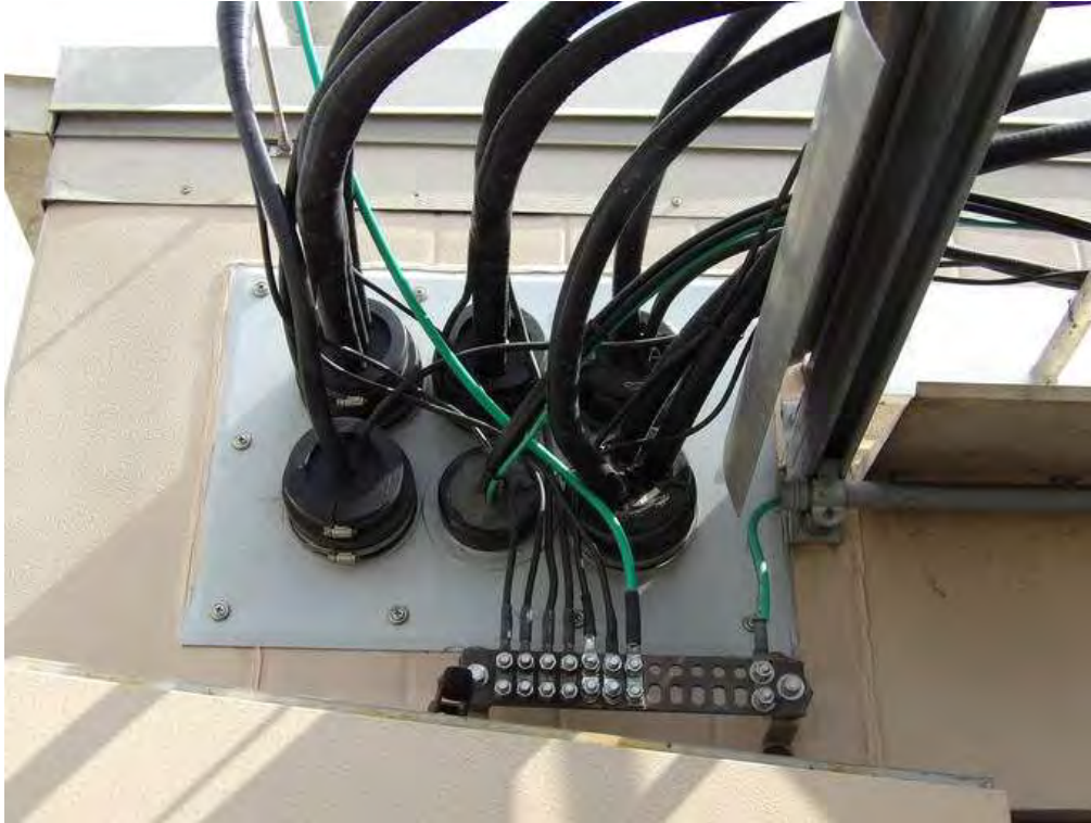
Antenna Exterior Entry Port
