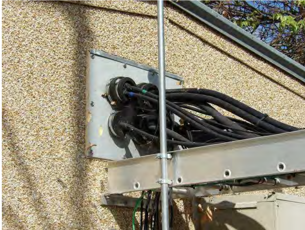
Antenna Exterior Entry Port
