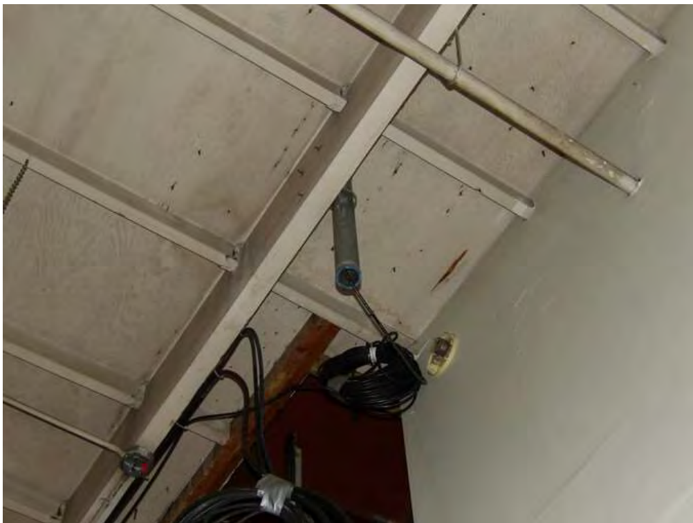
Antenna Cable Interior Entry Port
